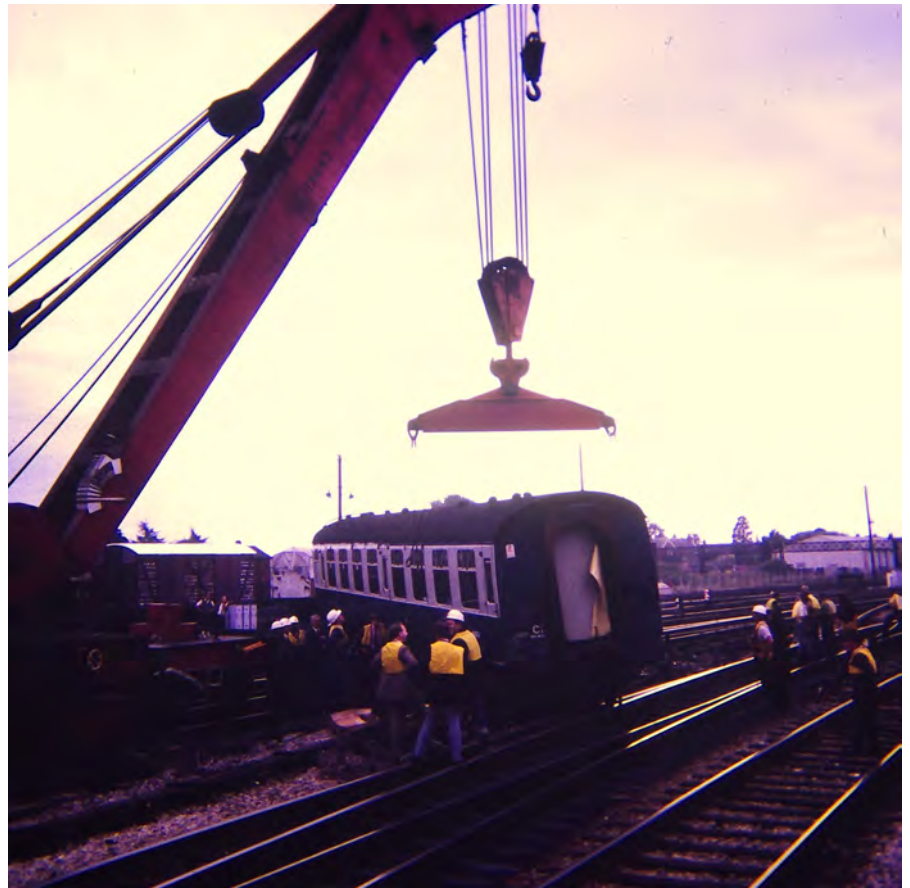
Photo: The lift is about to start. The crane will lift the coach at the derailed end, then slew to the left and place the derailed bogie back onto the down relief line where 25052 is ready to take it away and clear the line. David Hartland
