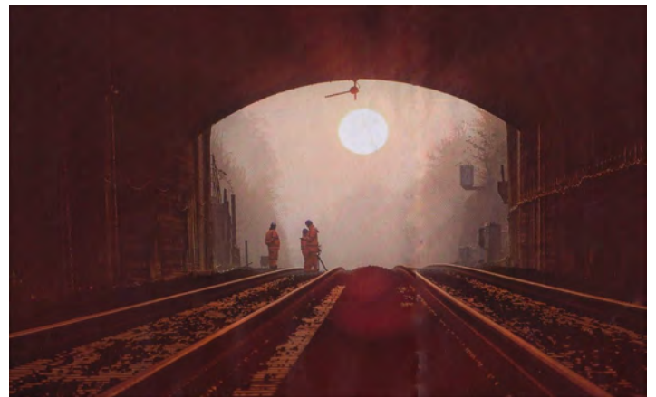
Eastern Portal of the tunnel at 6.30 on 9th April 2017. The sun is shining into the tunnel, and note that it is above the top of the cutting, but not by much. Adam Scott Images
