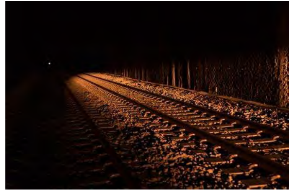
View into the tunnel and the sun's rays are failing to reach the far end. Adam Scott Images
