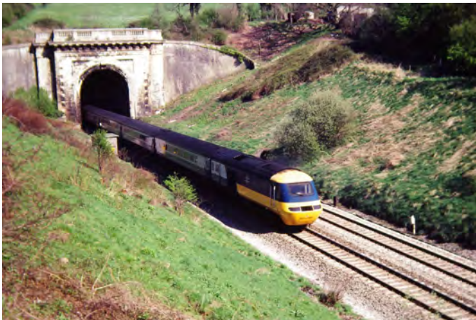
Up HST entering West Portal of Box Tunnel David Hartland
